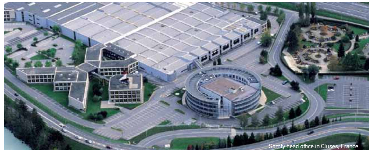
Somfy head office in Cluses, France
